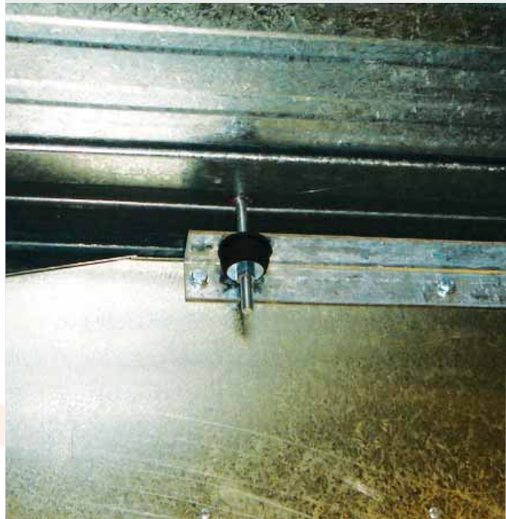
Figure 14(b). Optional rubber mount installed
